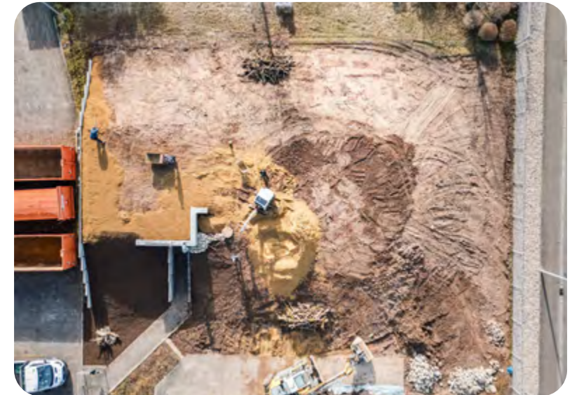
Construction phase of a new NABU-compliant planting mound
