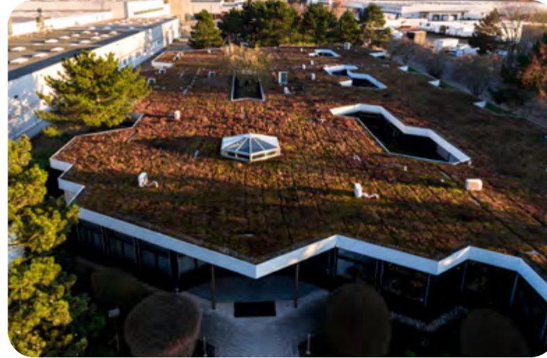
Green roof and garden
