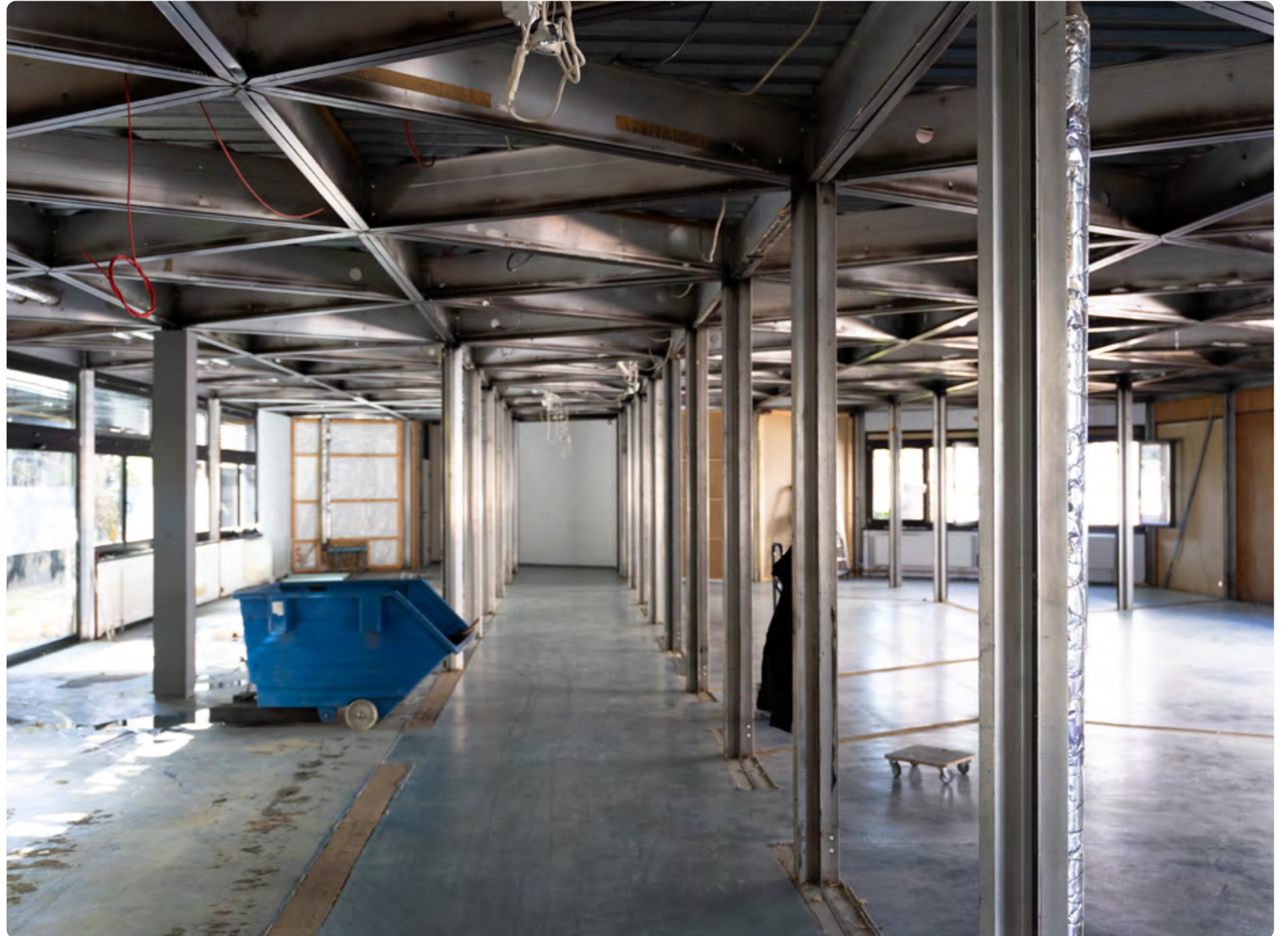
Renovation of the interior of the administrative building
